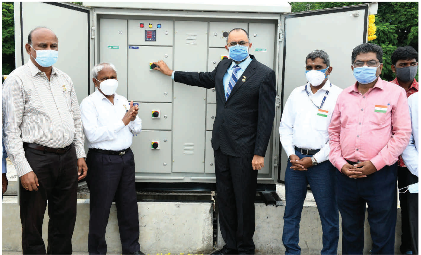
Illumination Facility at Coal Berths 3 & 4
