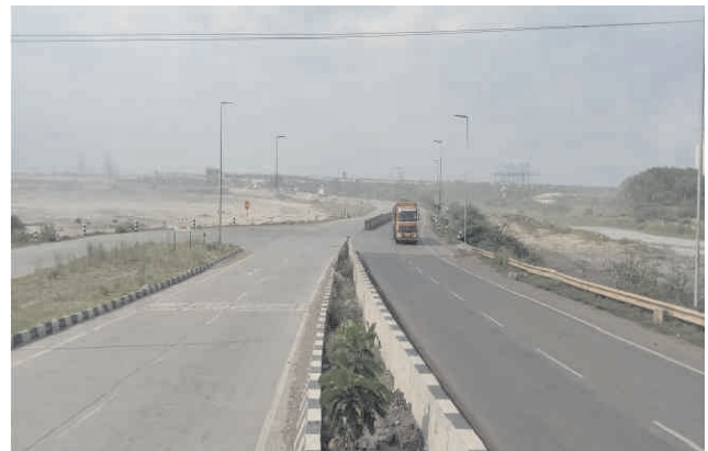
Southern Port Access Road
