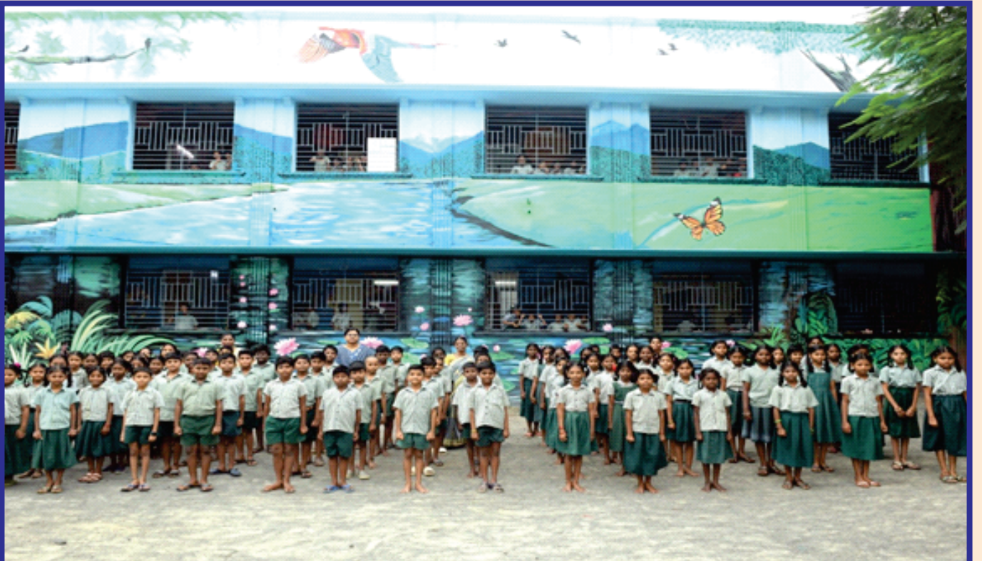
Construction of Classroom Building at GCC Middle School, Padasalai Street, Manali under Nammaku Namme Thittam
